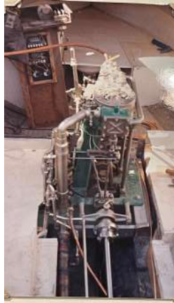
Aft view of engine while being installed
