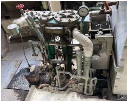
Engine—Port side Note hot well between engine and boiler
